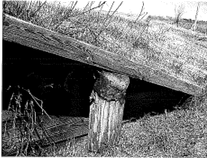
. Sample AB-1. Asbestos sample from wing wall pile NE corner of Bridge.
