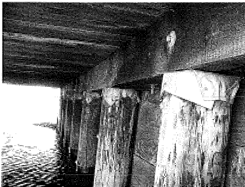
South abutment showing Sheet metal pile caps. Typical.
