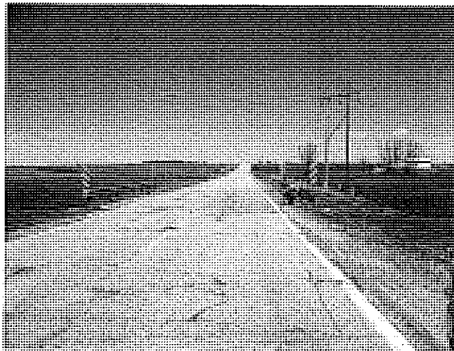
South approach to bridge looking North.
