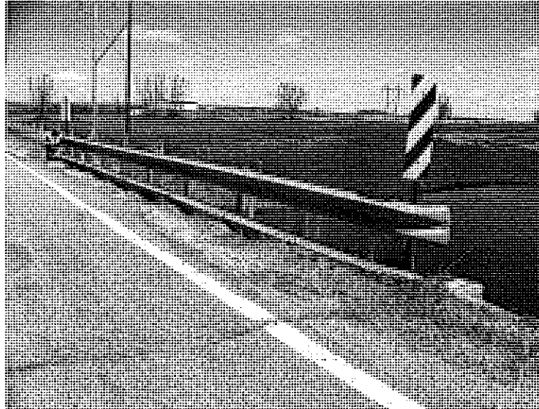
W-beam guardrail on East side of bridge.
