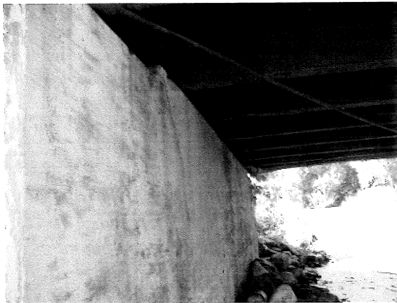
C-I-P concrete abutment at South end of bridge.
