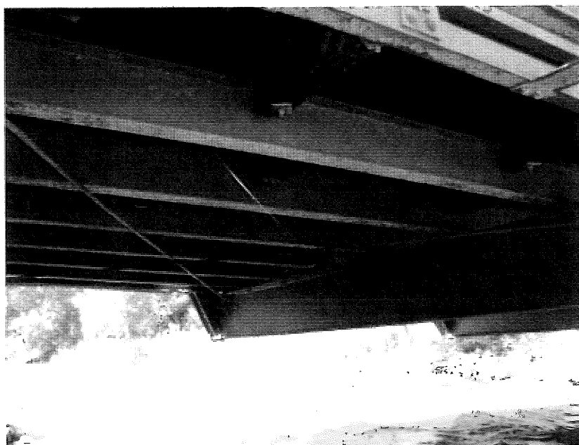
Under side of deck showing timber deck on steel stringers.
