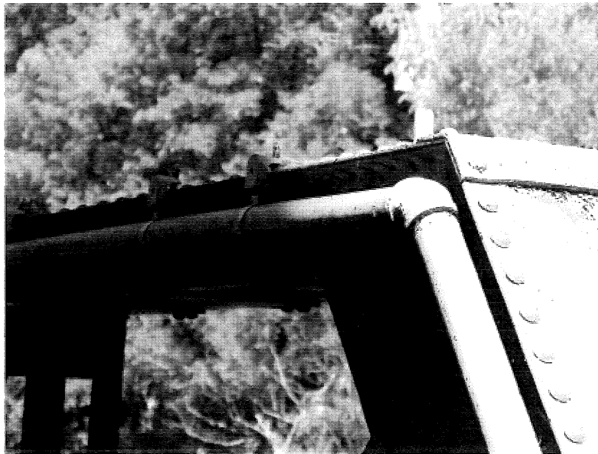
Conduit on upstream side of bridge.
