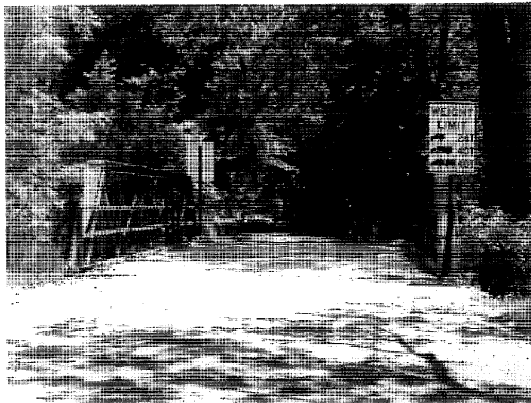
South approach to bridge looking North.
