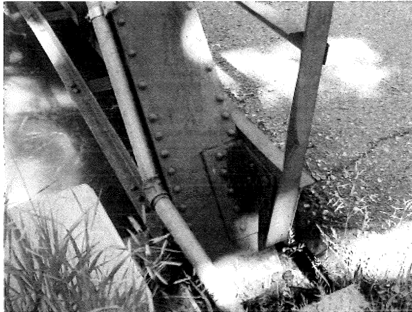
Possible utilities in conduit on upstream side of bridge. Owner unknown.
