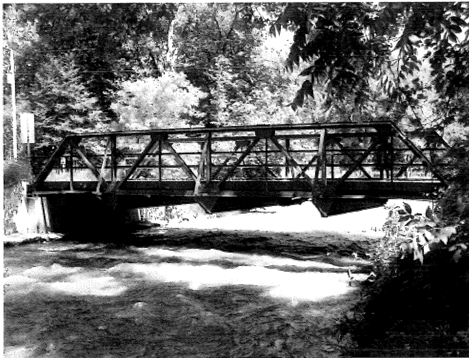
East side of bridge.
