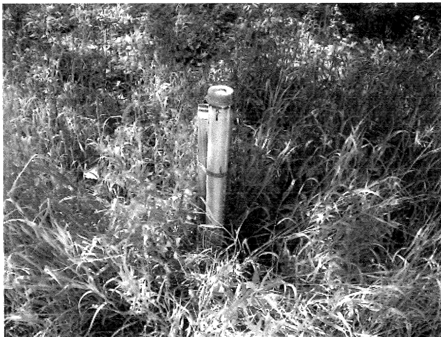
Stand pipe installation on West R/W line approximately 100' North of bridge. Owner and function unknown.
