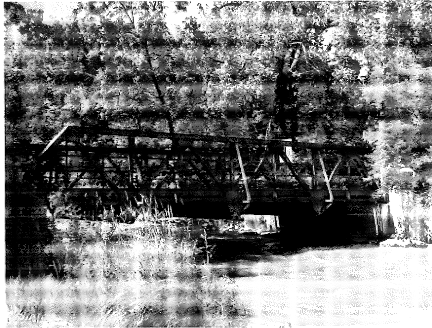
West side of bridge.
