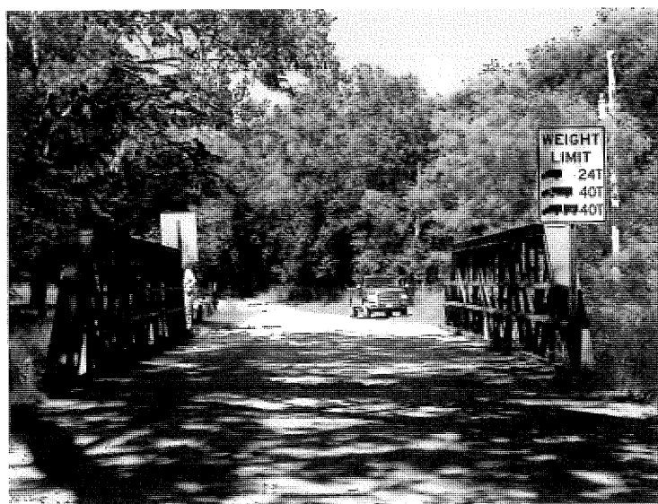
North approach to bridge looking South.
