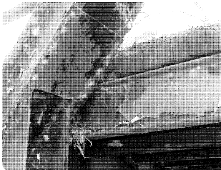
Sample LP-4. Lead paint sample from gusset plate at NE corner of bridge.
