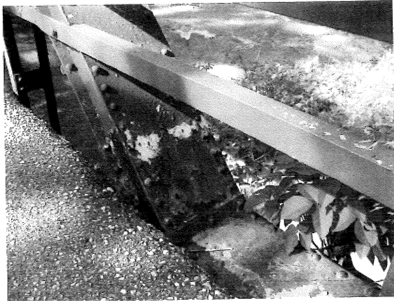
Steel angle iron railing affixed to truss members.
