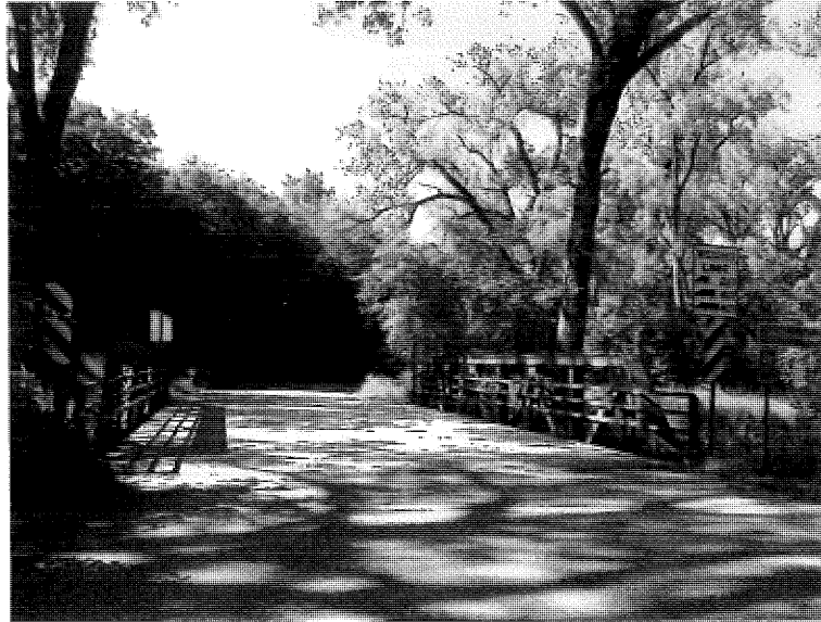
South approach to bridge looking North.
