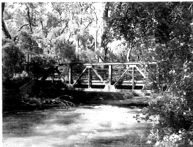
West side of bridge.
