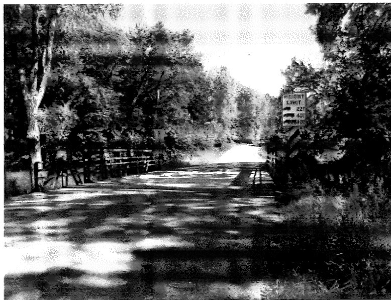
North approach to bridge looking South.
