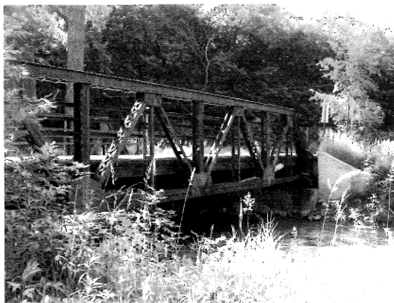
East side of bridge.
