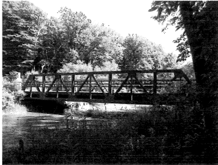
East side of bridge.
