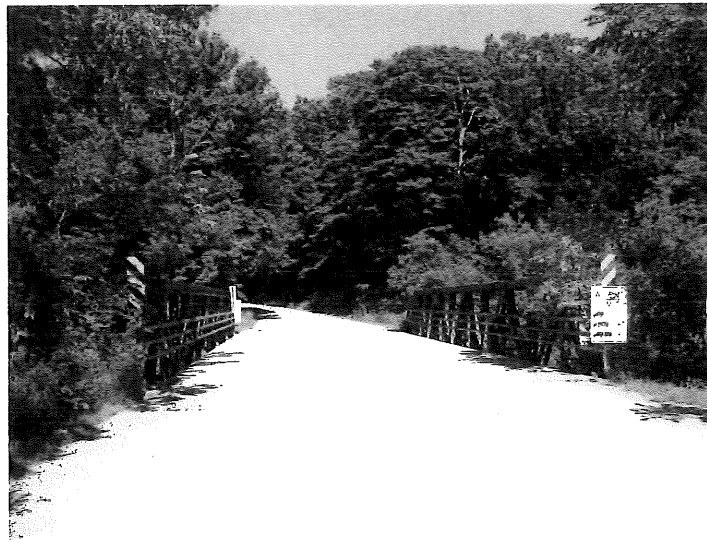
North approach to bridge looking South.
