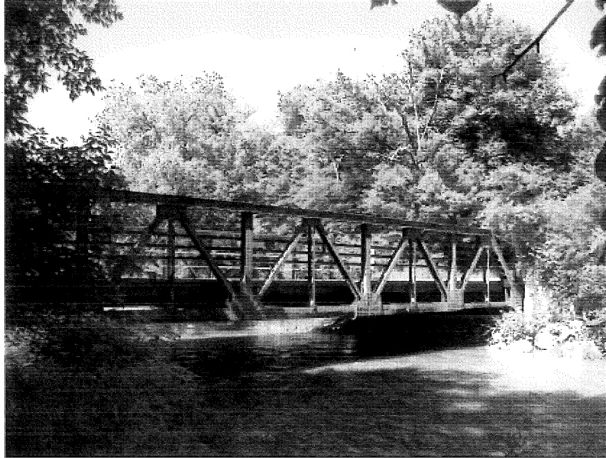
West side of bridge.
